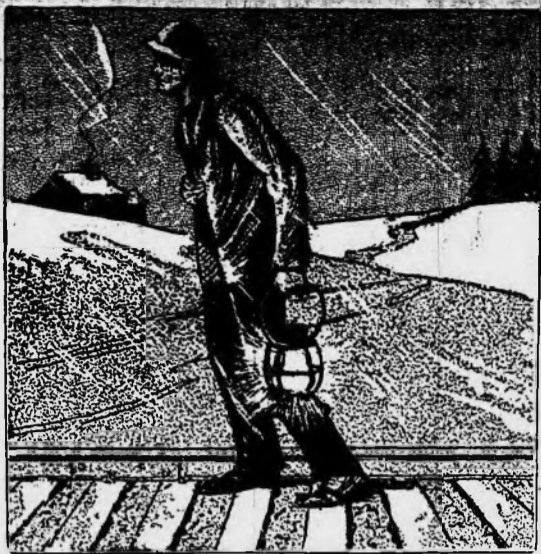
Watching the Ties and Rails.
