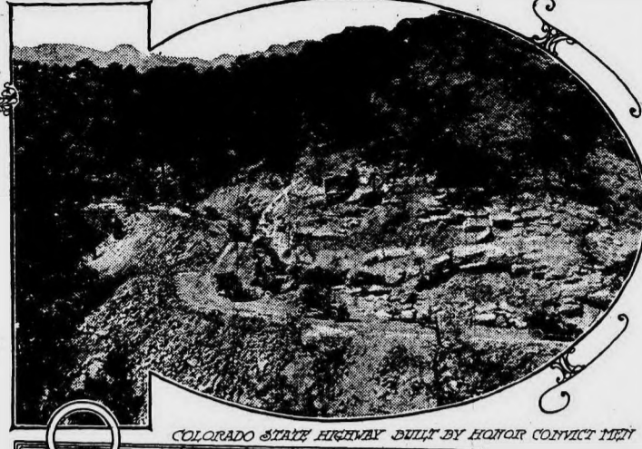
COLORADO STATE HIGHWAY BUILT BY HONOR CONVICT MEN
