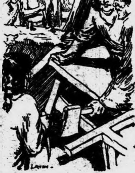
The Door Crushed In.
