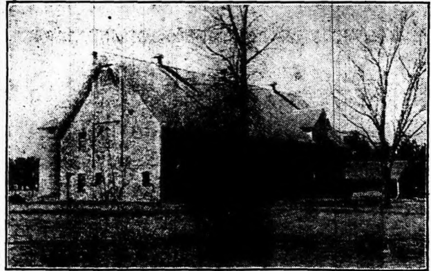
Main Portion of Dairy Barn at Iowa State College. (Planned by the Writer.)
