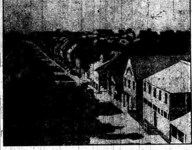
View of One of the Principal Streets Leading to Harbor. Great Damage and Fire Which Followed in This Section.
