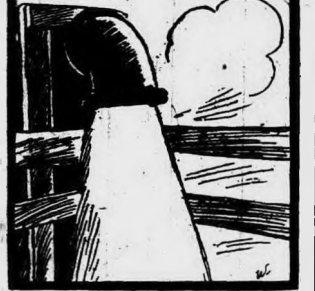
One of the Wells Which Furnishes Over a Million Gallons a Day.
