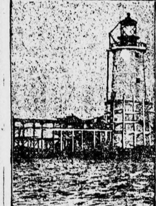
Ram Island Lighthouse. It looked just before the staging was removed.
