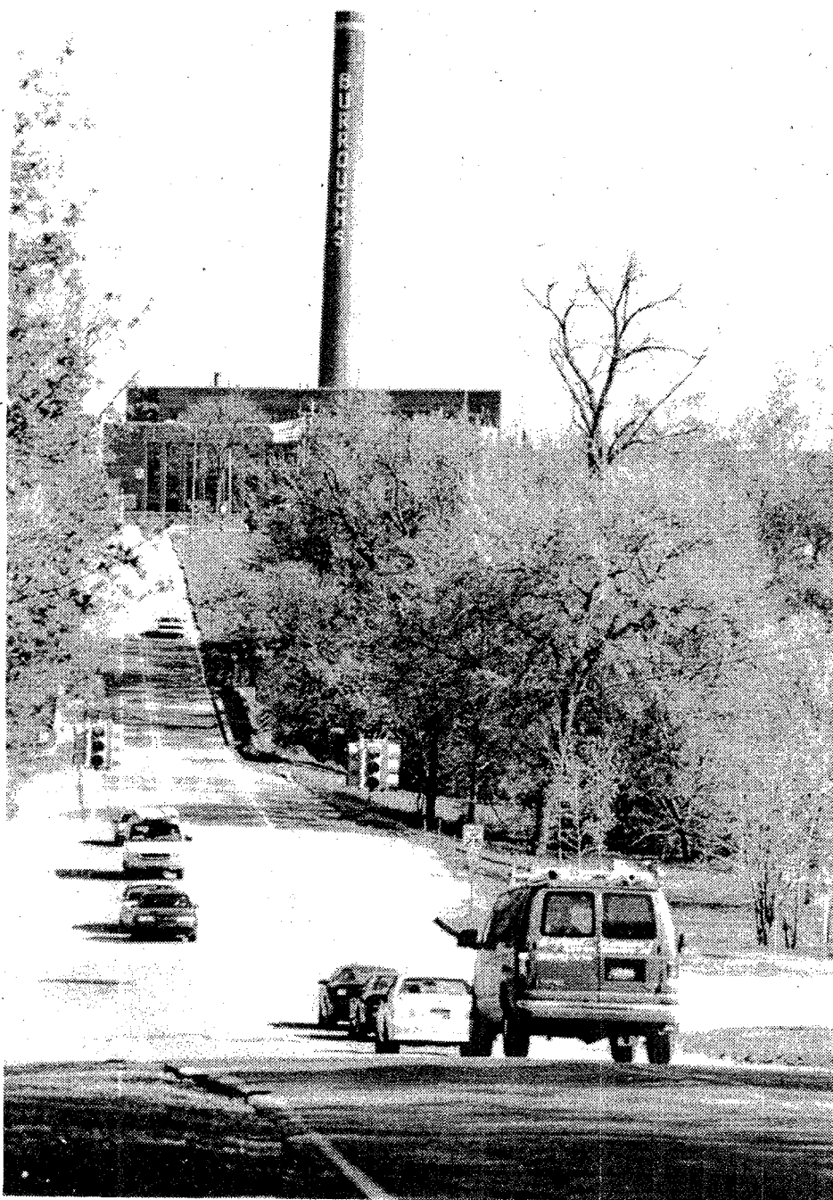
A sight associated with the drive into Plymouth for more than 60 years, the brick Burroughs smokestack will be taken down this summer. (Crier photo by R. Alwood, Jr.)
