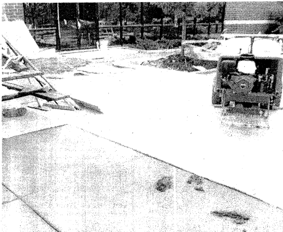
Tracks through the wet cement show the panic as employees of Johnson Controls fled their offices after hearing gunshots in their offices Monday. One observer said, "Here's the company trying to make this a better place for employees — building a patio and all — but no one can make this or anyplace absolutely safe." (Crier photo, R. Alwood, Jr.)
