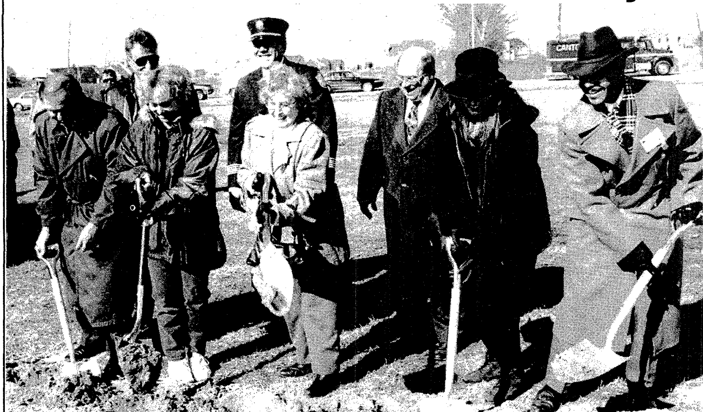
Canton officials broke ground on the 15,000-square-foot, $4.2 million fire station one and fire headquarters. The building will be located next to the Canton Administration Building. (Crier photo by R. Alwood Jr.)
