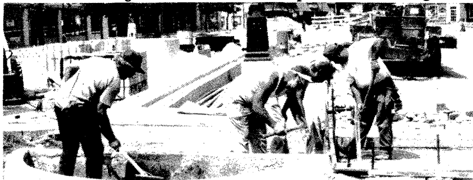
Work on Plymouth's Streetscape is nearly complete. (Crier photo by R. Alwood Jr.)
