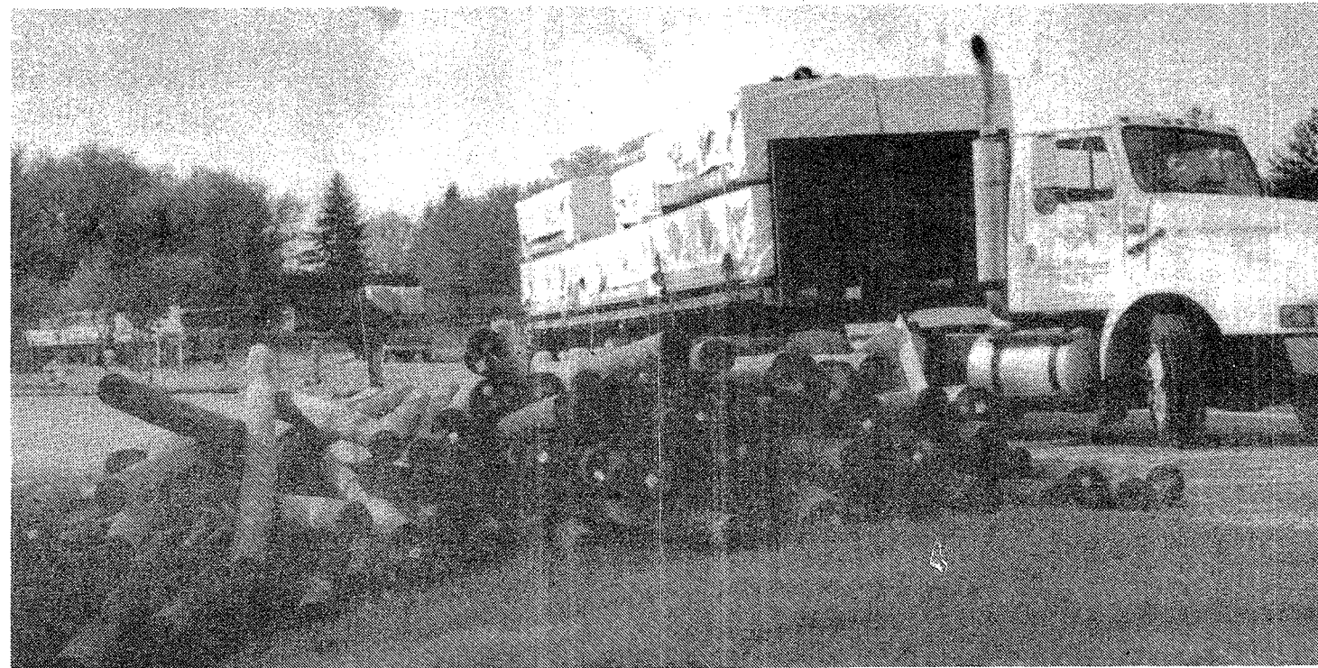
Biewer Lumber Company of St. Clair brought in the lumber that will be used for the long-awaited Plymouth Playscape project that officially began today at Plymouth Township Park. (Crier photo by Peter Broderick)
