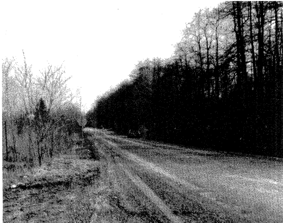
The paving of Koppernick road east of Haggerty would be one of the first projects undertaken by Canton if the road millage passes on the April 18 special election. (Crier photo by Craig Breil)
