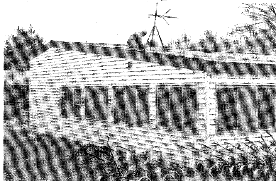
The Hill Top clubhouse (above) has been condemned since last fall, and a new proposal by golf course operator John Jawor calls for him eventually building a new facility in exchange for a two-year lease. (Crier photos q Lukasik)
