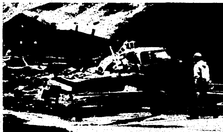
A utility official investigates the scene which caused approximately $2.5 million in damages when a building exploded and collapsed Friday morning. (Crier photo by Steve O'Leary)
