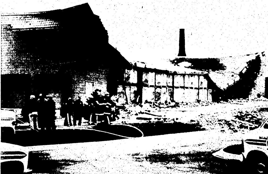
Fire officials survey the scene within a half-hour after an explosion destroyed the Cygnet Automated Cleaning company Friday morning. (Crier photo by Steve O'Leary)
