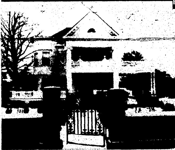
The outside of the City's Wilcox House was renovated last year. Work on 60 apartments around it was delayed, however. (Crier photo by Eric Lukasik)
