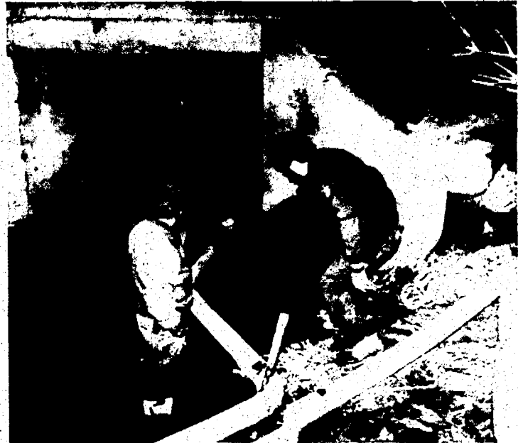
MPC crews lay a boom in front of the pipe where gasoline poured into Sly Drain most of Friday and Saturday. One of the crew points to the culprit. (Crier photo by Philip Tardani)
