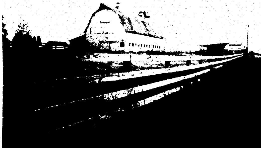
A barn on Curtis Road (Crier photo by Chris Farina)
