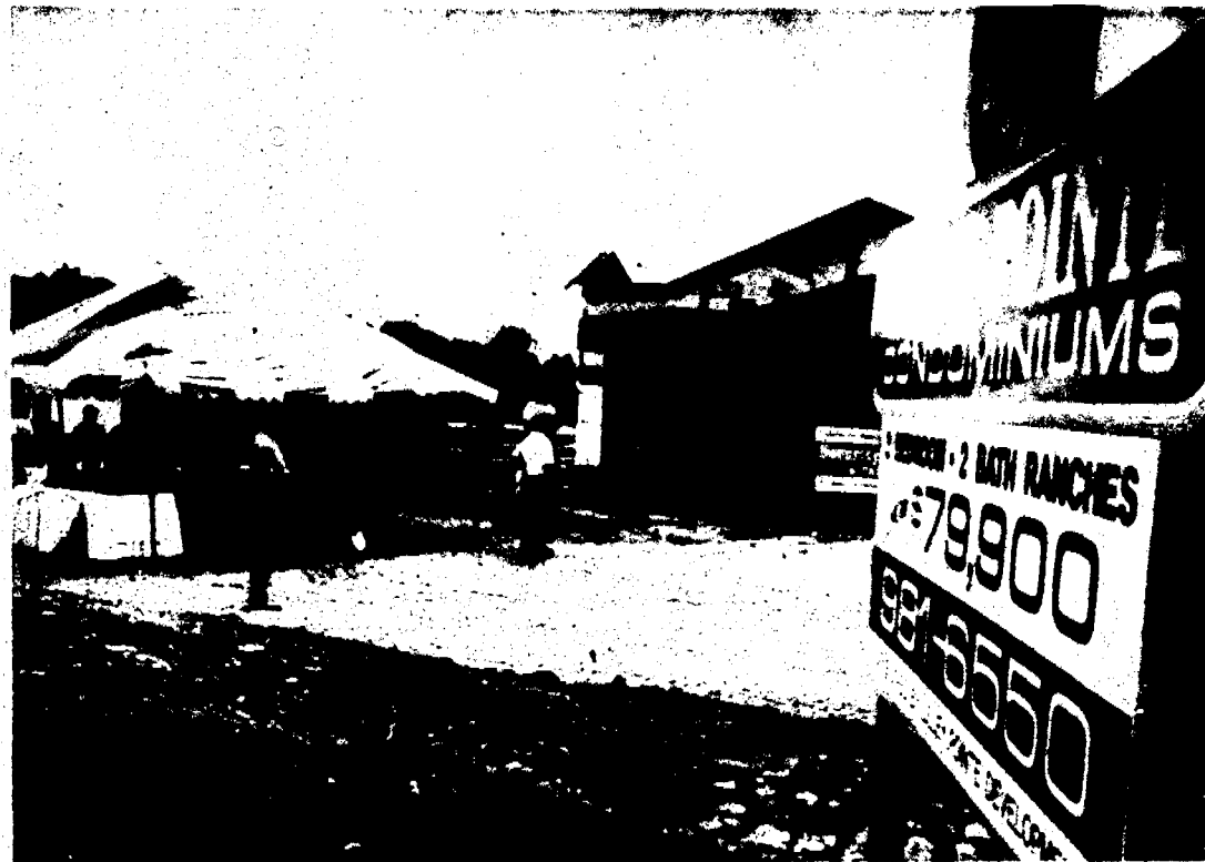
Ground has been broken for a new condominium project in Canton last week. The Lilley Pointe condo project is the township's largest such development.
