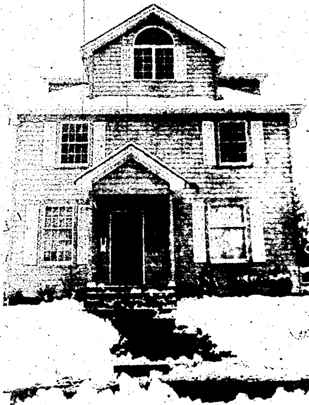
The outside of the house, built in 1910, was also completely redone.
