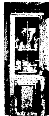
THESE DESIGNS for kitchen cupboards use lazy-susans and the insides of doors. At upper left is a "wastebasket drawer."
