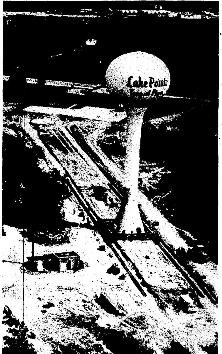
THE LAKE POINTE WATER TOWER was moved to make way for M-14, which was built in 1973. Along with the Lake Pointe area, sections of Old Schoolcraft, Beck and other roads were affected by construction of M-14. Shearer Drive, east of Sheldon Road, was completely removed. (Crier photo)
