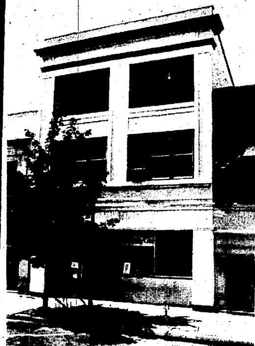
THE COMMUNITY CRIER today at 821 Penniman Avenue. Its publishing division, COMMA, is located in the other end of the building at 345 Fleet St.
