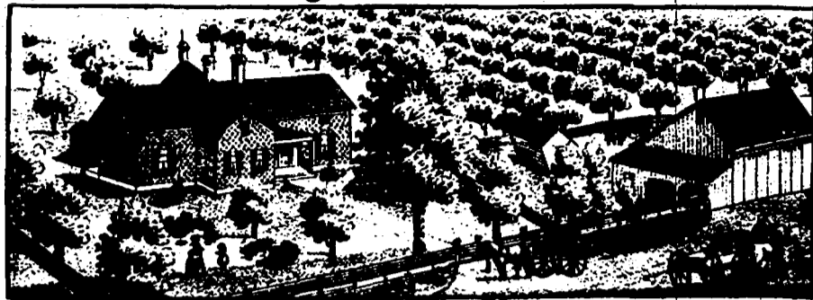
LOCATED NEAR SHELDON and Warren roads, the Pattengell farm appeared in the 1876 Wayne County Atlas.
