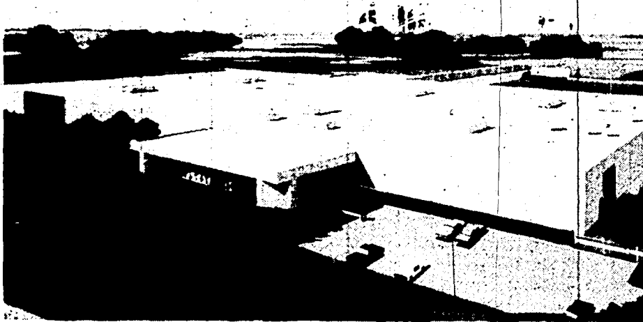
THE FORMER PRECISION SPRING PLANT soon to be occupied by Draw-Tite, Inc. in March.
