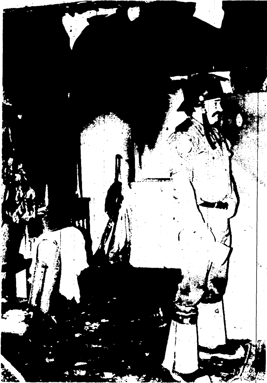
FRIDAY'S EXPLOSION ripped through the Canton residence on Pointe Street causing extensive heat and smoke damage. Above, Canton Firefighter Claude Gersky surveys the damage shortly after the explosion occurred.
