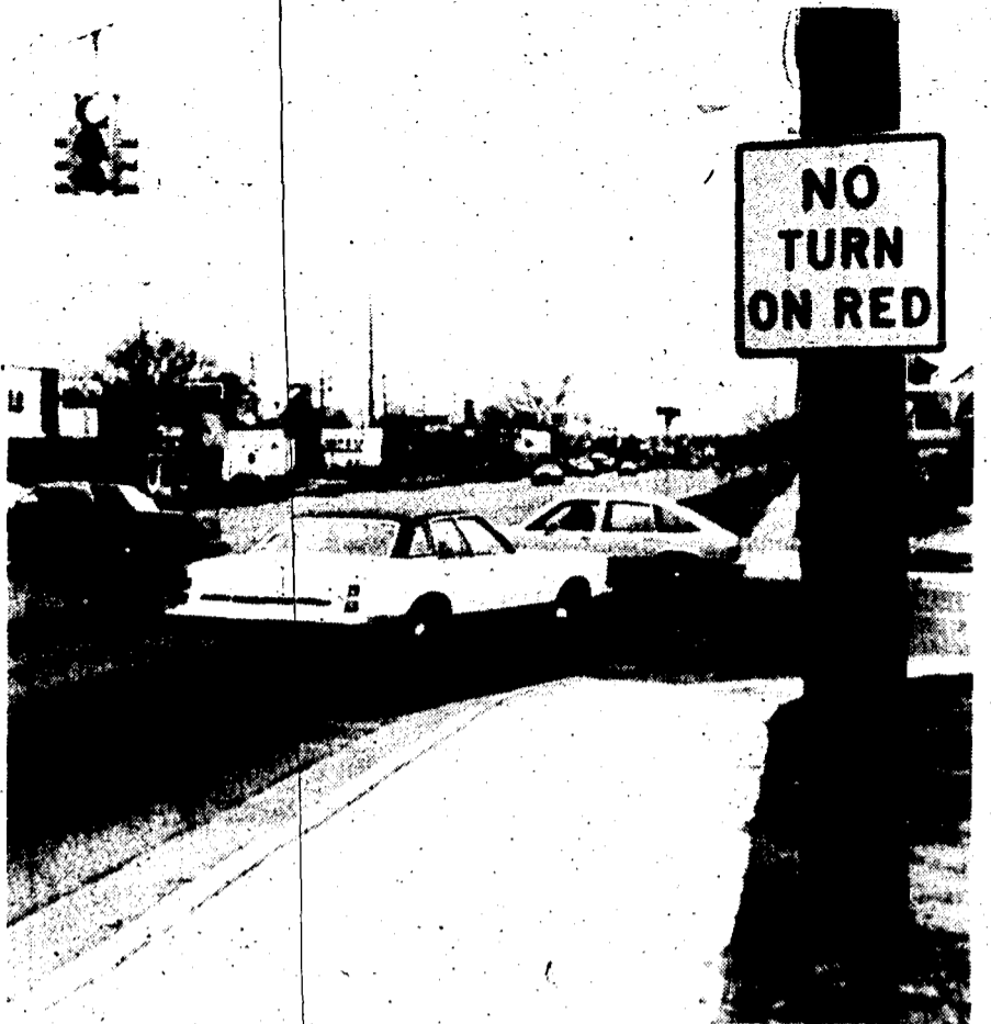
DRIVERS CAN NOW turn left onto Main Street from Ann Arbor Road on a "protected" left turn arrow. A "No Turn on Red" sign on the northeast corner of the intersection is too far from the corner, according to the Plymouth Police, and some drivers, like the one above, illegally turn right on red because they don't see the sign. (Crier photo by Rick Smith)
