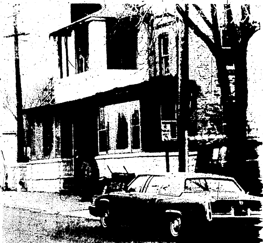
THE OLD VILLAGE INN was more than 50 per cent destroyed in the Jan. 5 blaze that claimed one life, says Plymouth City Engineer Ken West. That means that if the rooming hotel is to be rebuilt, it must be totally brought up to code. Hotel owner Eugene LaBlanc (whose car is shown parked in front of the Inn) says he wants to rebuild. (Crier photo by Rick Smith)
