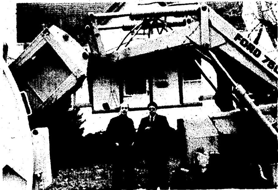
"THE CLAW" deposits a load of wet leaves in a truck stopped along a Plymouth street as DPW Superintendent Ken Vogras and City Manager Henry Graper look on. The hydraulic device attaches to a front-end loader and was purchased by the city to augment the existing leaf vacuum which is not designed to remove wet leaves. (Crier photo by Rebecca Beach)
