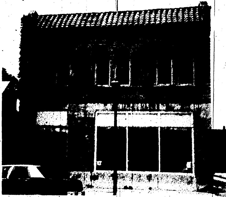
THERE ARE THE NEW quarters for Wade, Trim Environmental Group, Inc. The building, at 729 W. Ann Arbor Trail, has undergone extensive remodeling in past months to make room for administrative offices of the firm. (Crier photo)
