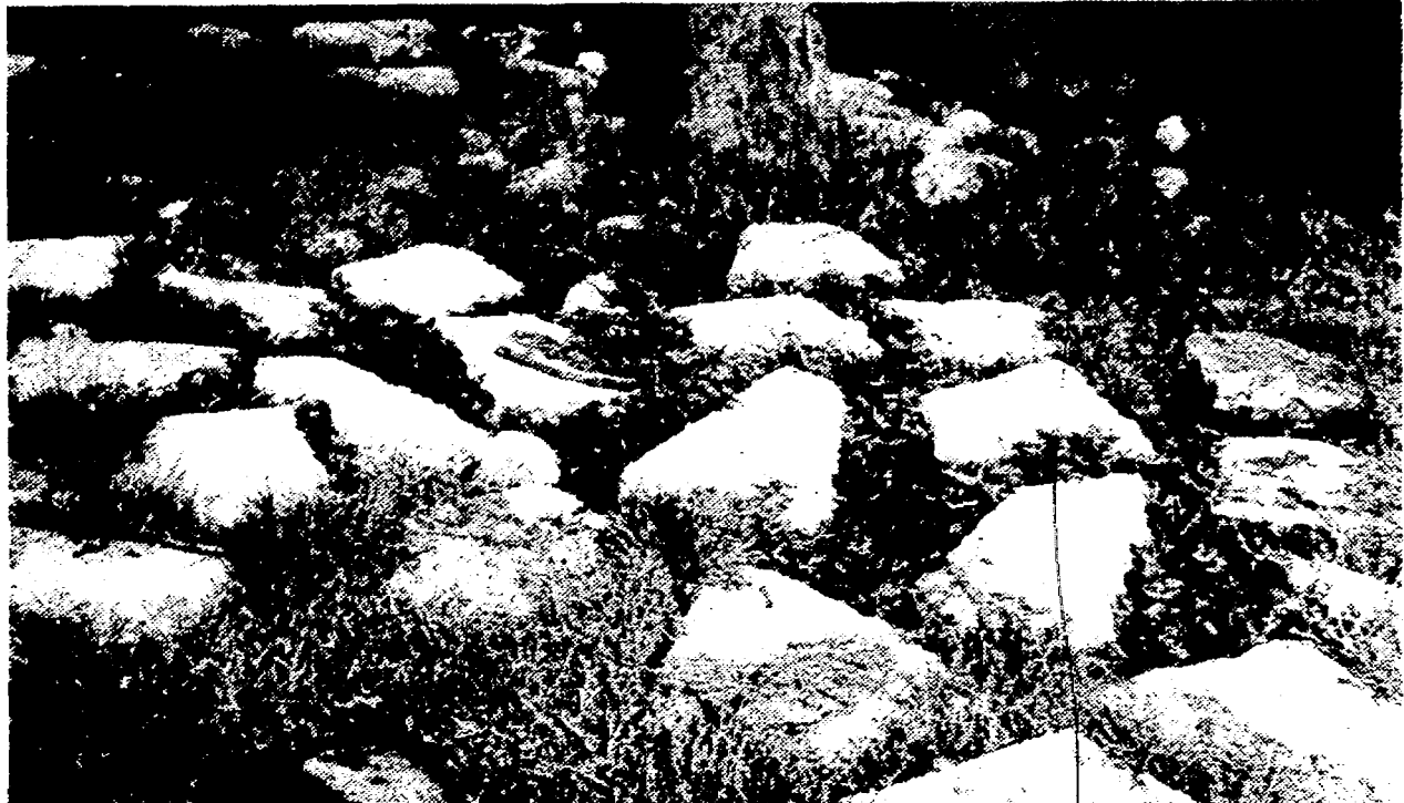
FANCY LANDSCAPING IT'S NOT. Backyards in Park Gardens Sub-division on the north side of Five Mile have lots of problems with septic tank effluent bubbling out of the ground. Backyards are soggy messes. This homeowner placed chunks of concrete on top of the quagmire.
