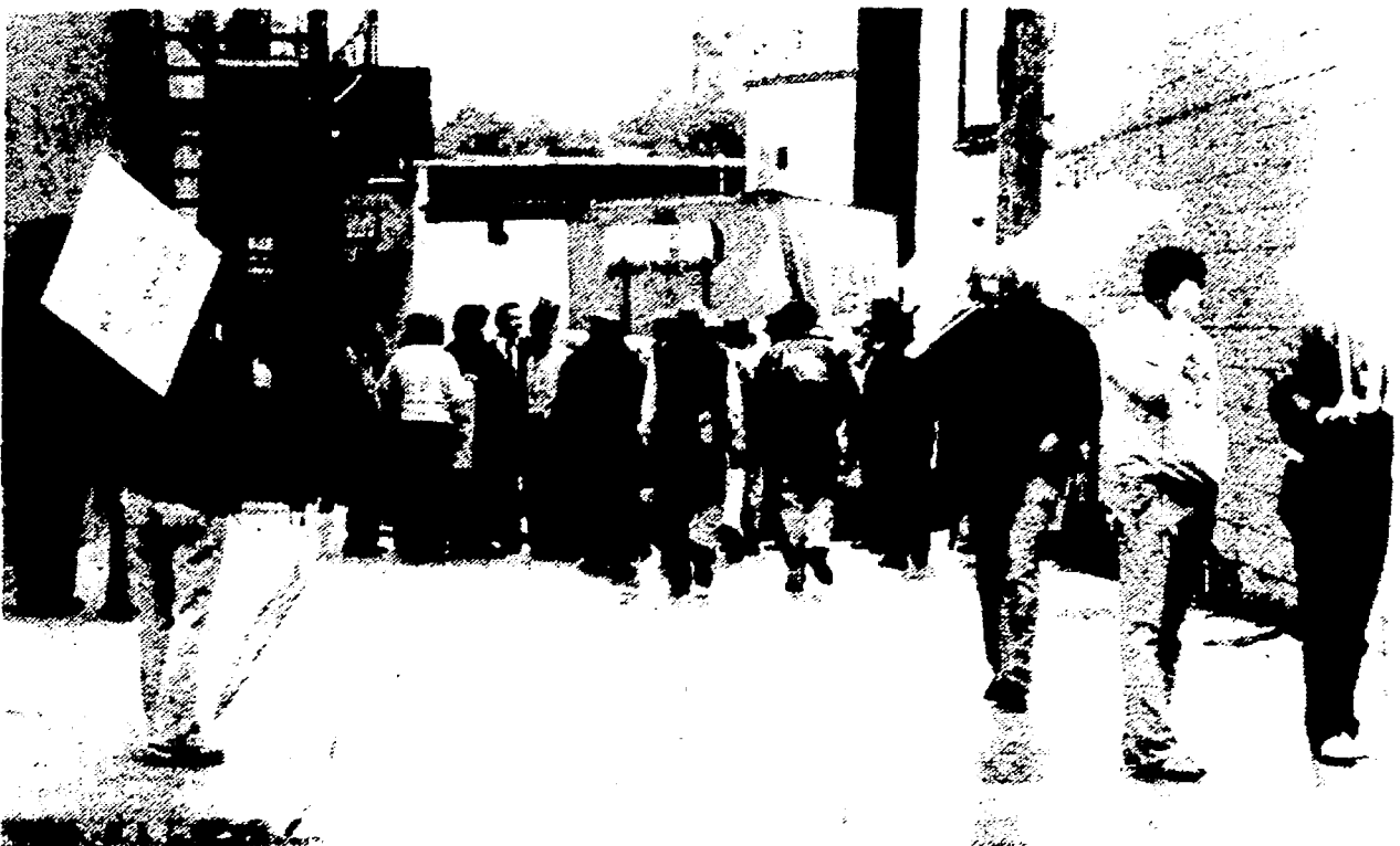
AMIDST THE PLUMBERS UNION pickets, general contractor Don Bidwell (in vest walking away from camera) surveys the situation on the Mayflower Hotel Annex - Wiedman Parking Lot project. The pickets shut down the project in their protest against Long Plumbing. (Crier photo by Robert Cameron)
