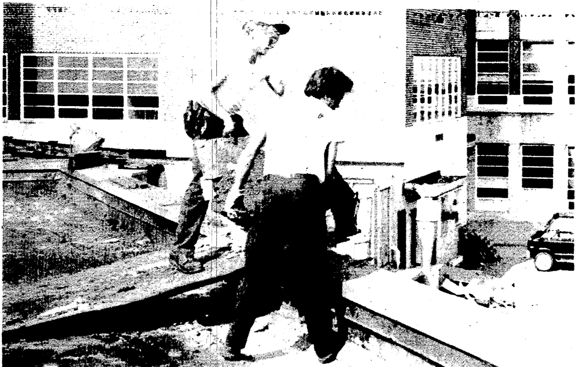
Fixing a hole where the rain gets in
