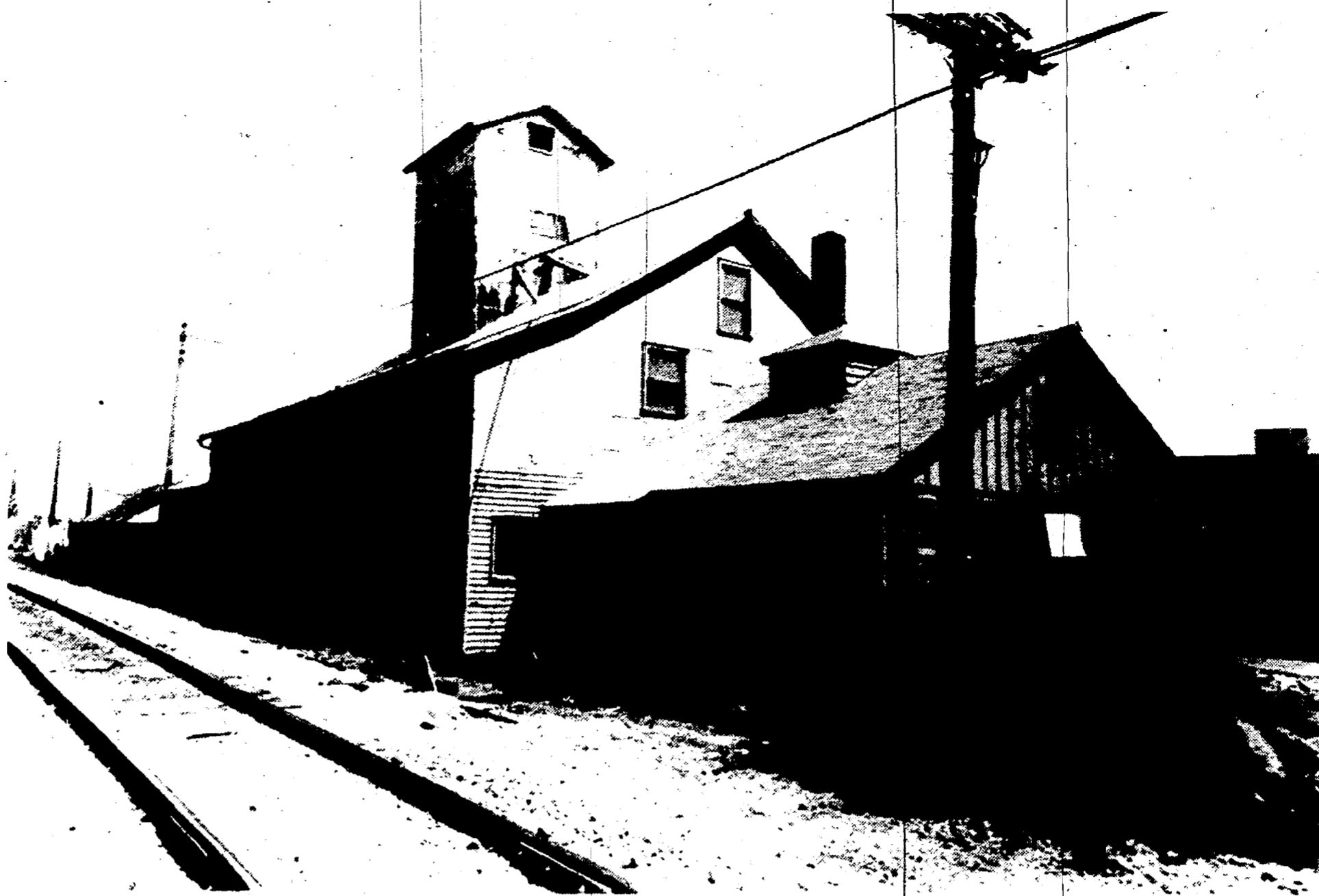
THE OLD MCLAREN bean mill at North Main Street will eventually have a brand new exterior and interior once owner Gene Glynn finishes the restoration project he and his crews are currently
