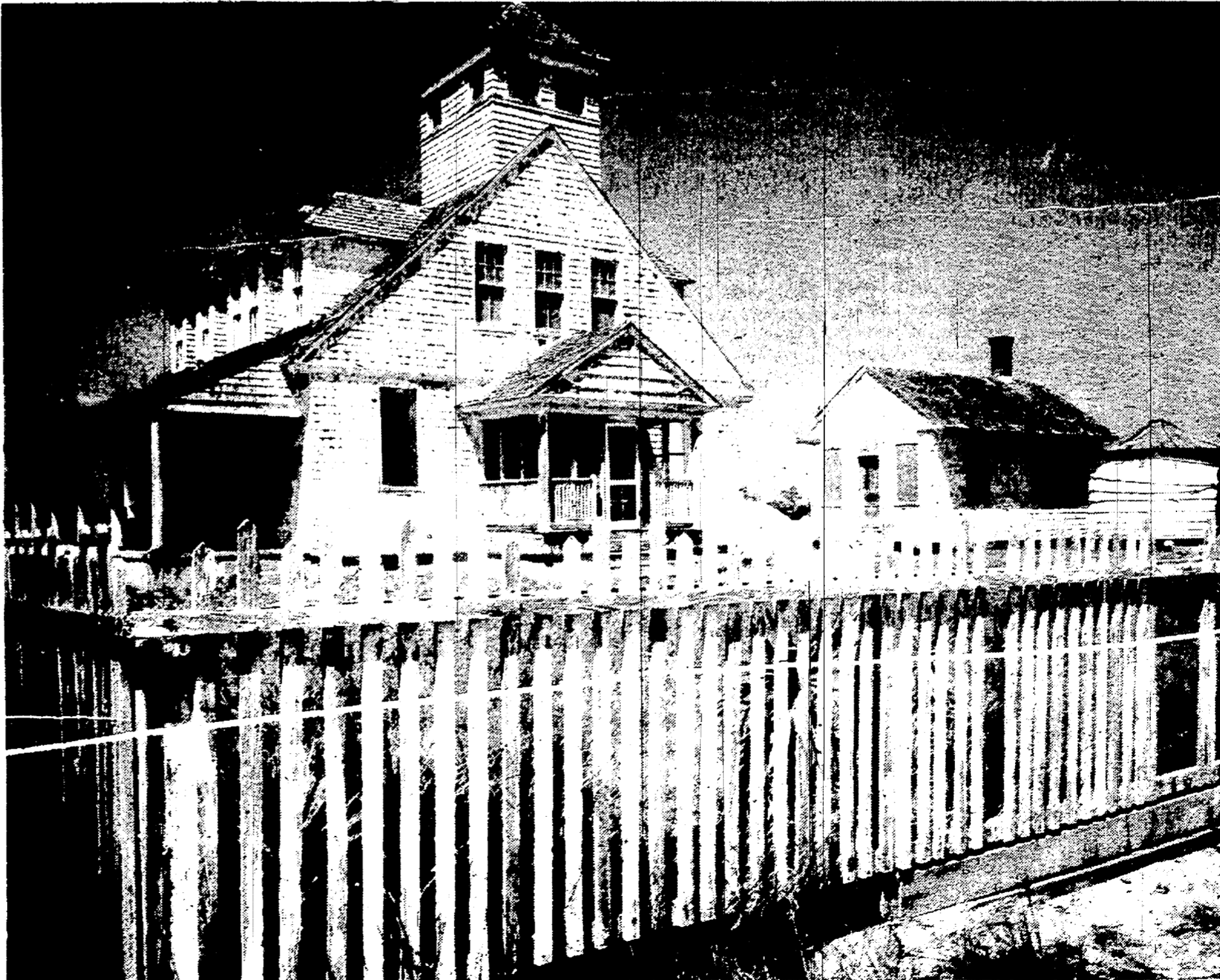
Chicamacomico Coast Guard Station, Outer Banks, North Carolina.
