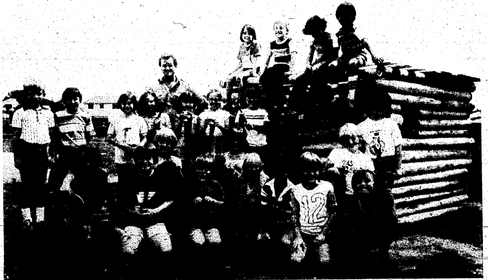
CONSTRUCTION OF this log cabin at the Isbister School playground started 10 weeks ago. After studying pioneer life, the students earned money through bake sales for the cabin, which cost $550.
