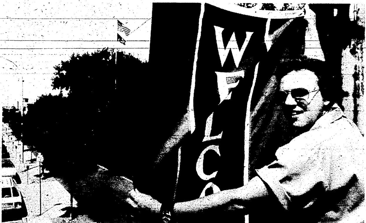
RICH RUSSO of the Plymouth Department of Public Works helps install one of the welcome banners for the GOP delegation on Main St.
