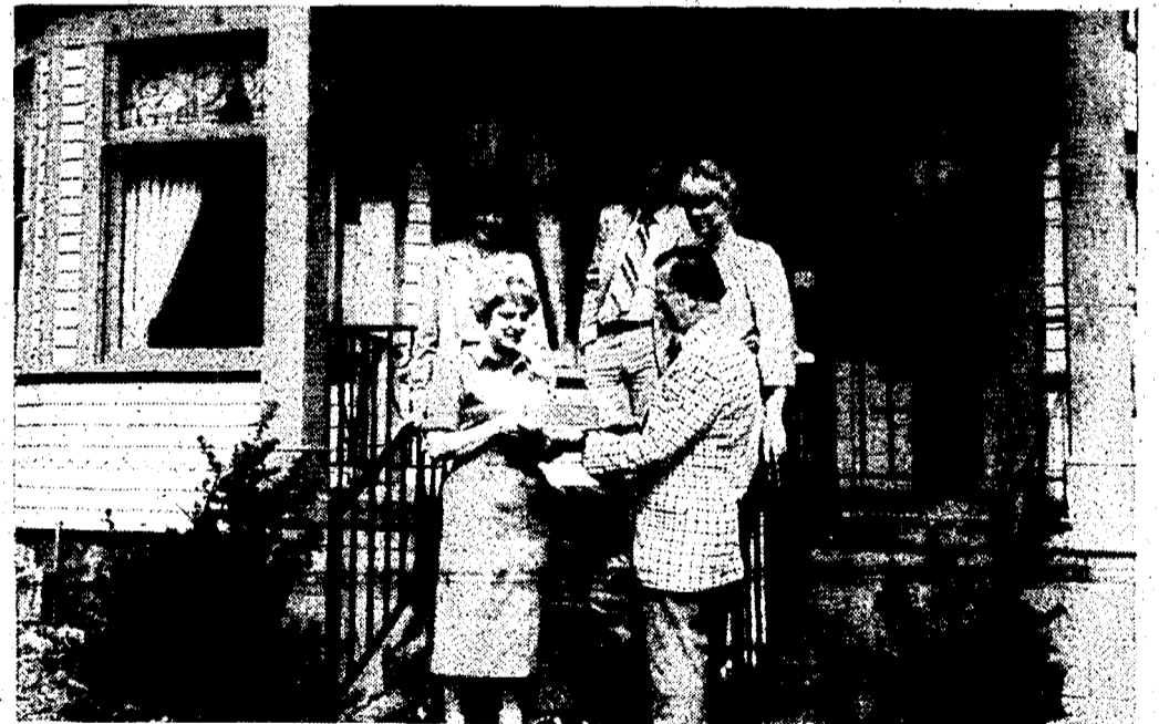
THE AMERICAN ASSOCIATION OF UNIVERSITY WOMEN honored the old Plymouth Hospital building with a Landmark award. Presenting the award was Mary Kehoe (left front) to Charles Reinhart, owner of the building. Watching the presentation were (from left) Susan Schrader, Ron Martin, and Donna Keough. (Crier photo by Phyllis Redfern)
