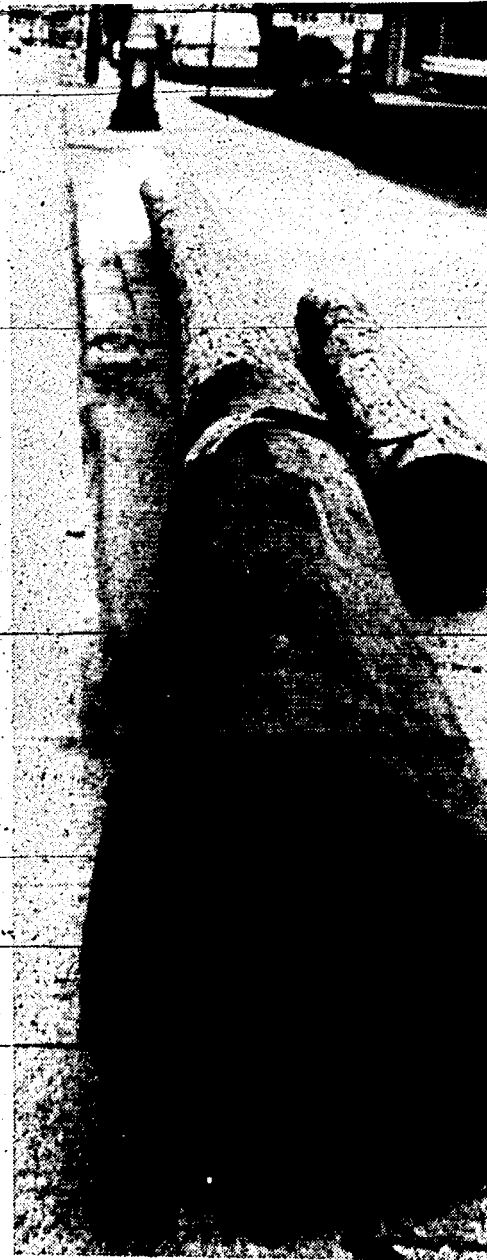
THESE UTILITY POLES have been lying, partially out into N. Main St., for more than a week. They pose a hazard for traffic in the right-hand lane if traveling close to the curb. Neither city police nor the DPW have taken any action to relieve the problem. (Crier photo by Robert Cameron)
