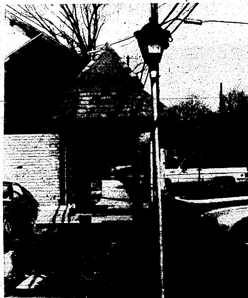
WORK IN PROGRESS in Old Village includes a wooden kiosk in the square between Mill and Starkweather streets that will feature the names and logotypes of Village shops. The 19th-century-style lamppost in front is one of about a dozen that have been installed in the past year. (Crier photo by Robert Kian.)
