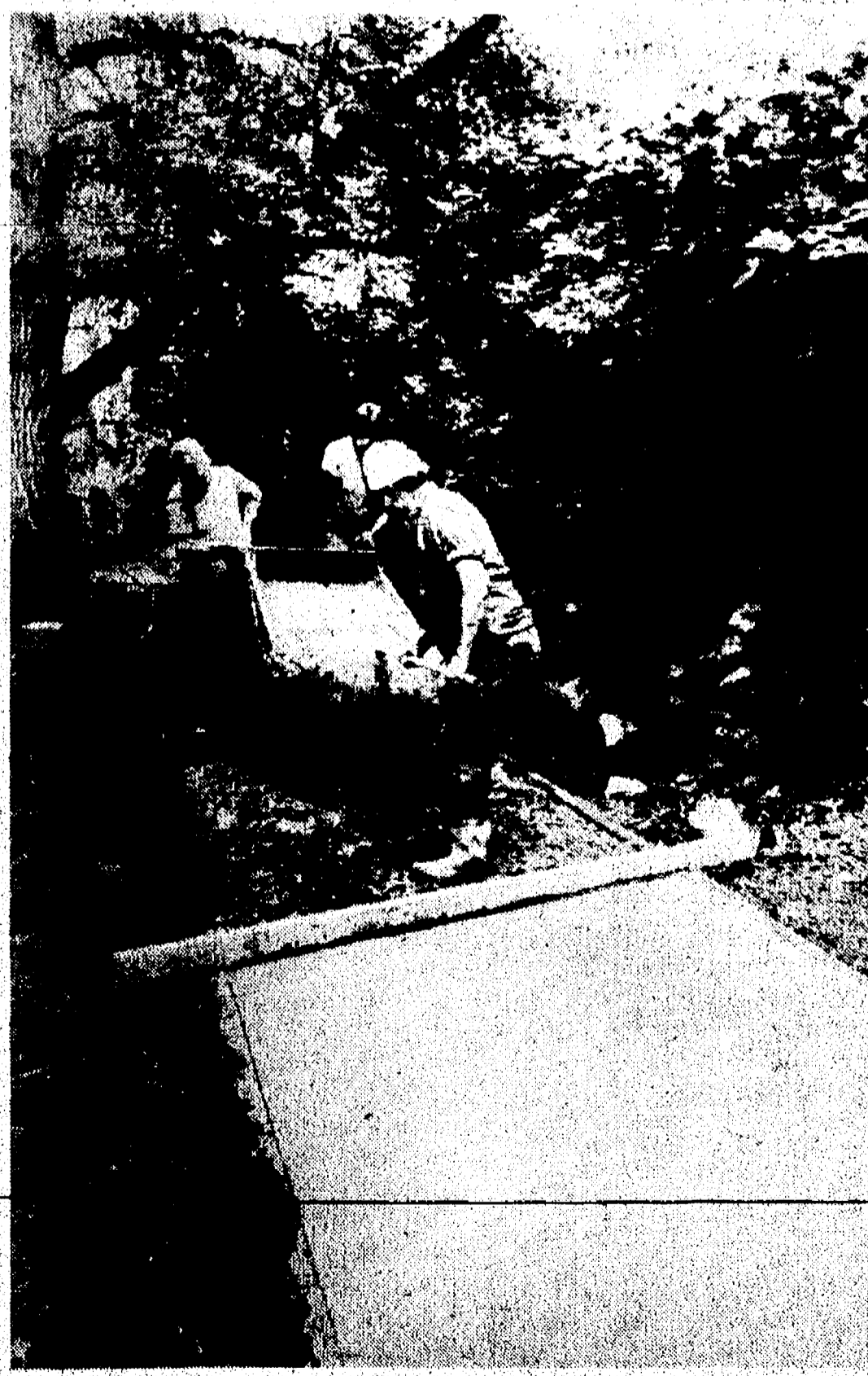
THE TONQUISH CREEK WALKWAY was underway last week as city workers started to pour concrete. When finished, the walkway will connect with Tonquish Creek Manor and also provide a bridge. (Crier photo by Brian Watkins).
