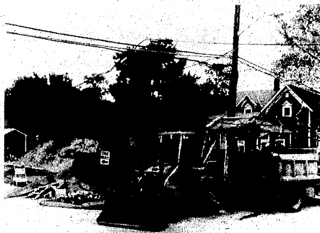
CONSTRUCTION IS WELL UNDER WAY in Old Village on a parking lot and a cobblestone courtyard. Builders hope to have the project completed in time for "Dearie Days" July 23. (Crier photo by Brian Watkins).
