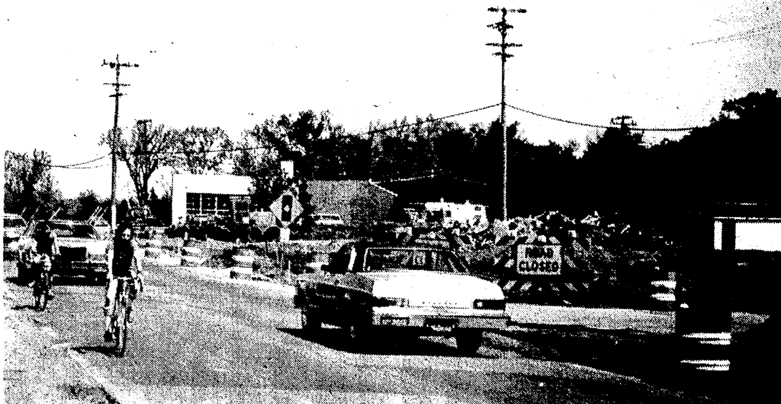
WITH CONSTRUCTION of the M-14 Expressway progressing, Northville Road is being rerouted. The new highway will pass just
