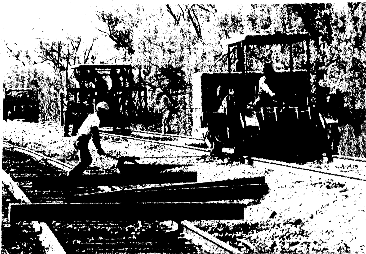
REPLACING THE GANDY DANCER. Crews which used to straighten railroad tracks and pack ballast, this C&O crew and machinery is already at work upgrading tracks in the Plymouth-Canton area. (Crier photo by Susan Sheiner.)
