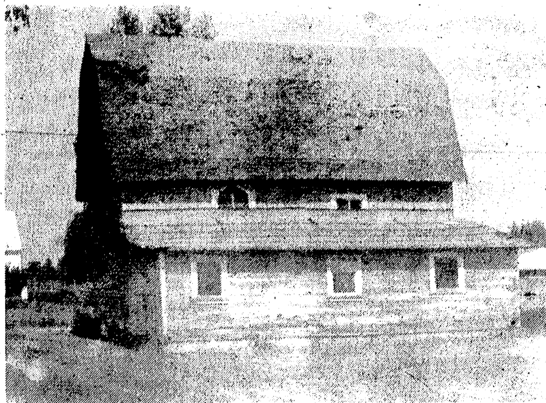
THE PENNEY FEED MILL as it appeared before its lean-to shed once used as a blacksmith shop was removed, will soon be torn down to make way for a new Canton street. The feed mill was a well-known business to many area farmers.
