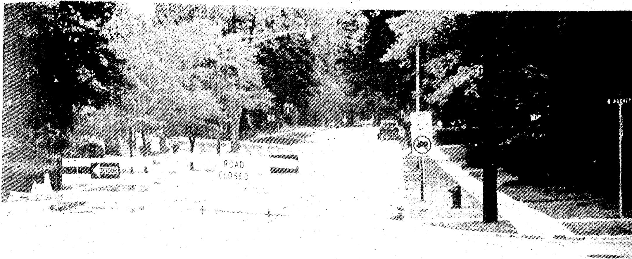
REOPENED YESTERDAY PG. 13 after barricades closed it to traffic for nearly a week was Church Street between Harvey and Pennington. Plymouth DPW workers closed the thoroughfare to repair buckled pavement near Harvey. (Crier photo)
