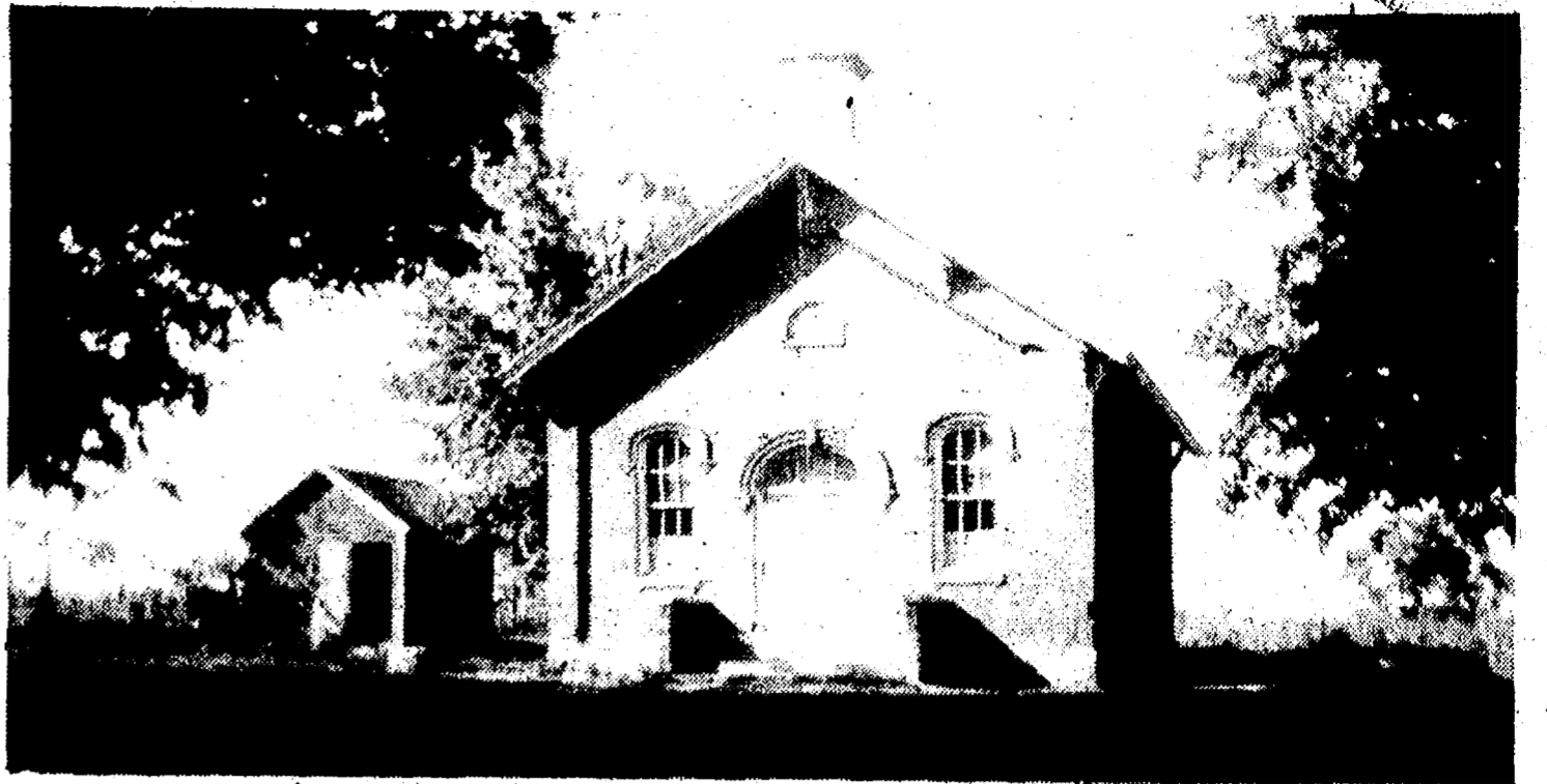
CHERRY HILL SCHOOL , known years ago as Fractional No. 1, was adopted by the late Henry Ford Sr. as one of his Greenfield Village Schools. Located in Canton at the corner of Ridge and Cherry Hill roads, the school was enlarged by Ford as a favor to the school board for allowing an indigent family's children to attend there. The school is now used by a church but belongs to the Plymouth School District. (Photo courtesy of Dorothy West)
